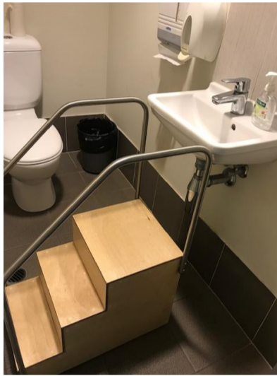
Stairs to Hand Basin
